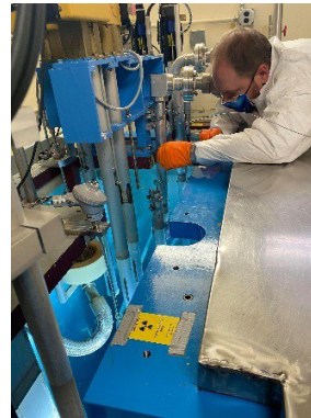
Installing SPND in the NRAD reactor.
