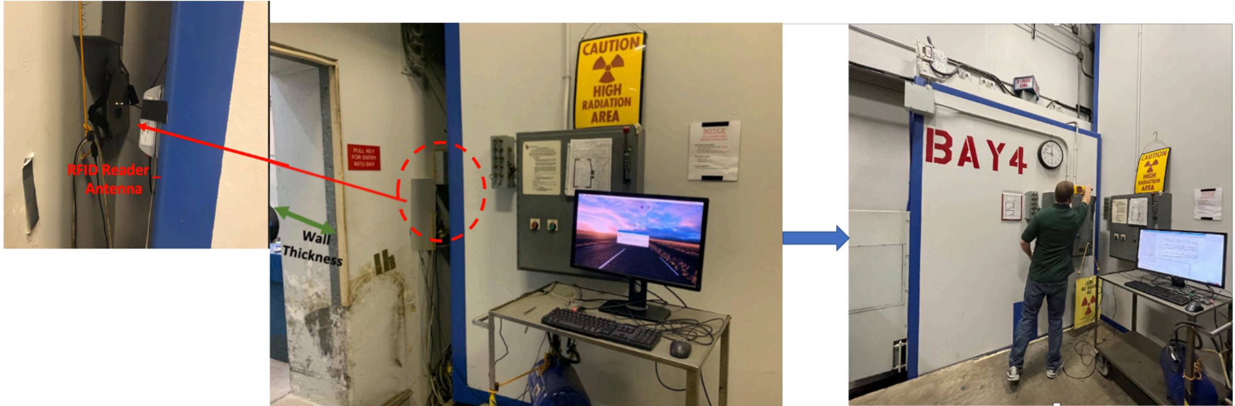
RFID antenna and reader outside the containment wall with open door to show the wall thickness
